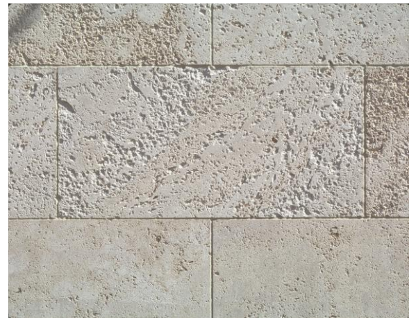
Travertine on the exterior of Nasher Sculpture Center
